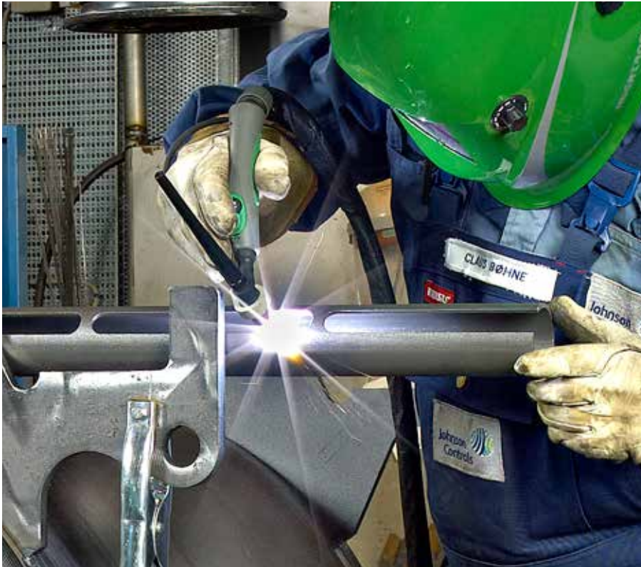
MMA in a V-joint
