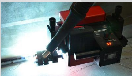
Torch placement on either side
